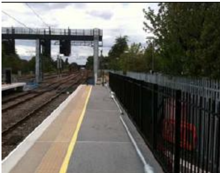
Bedford platform extensions
