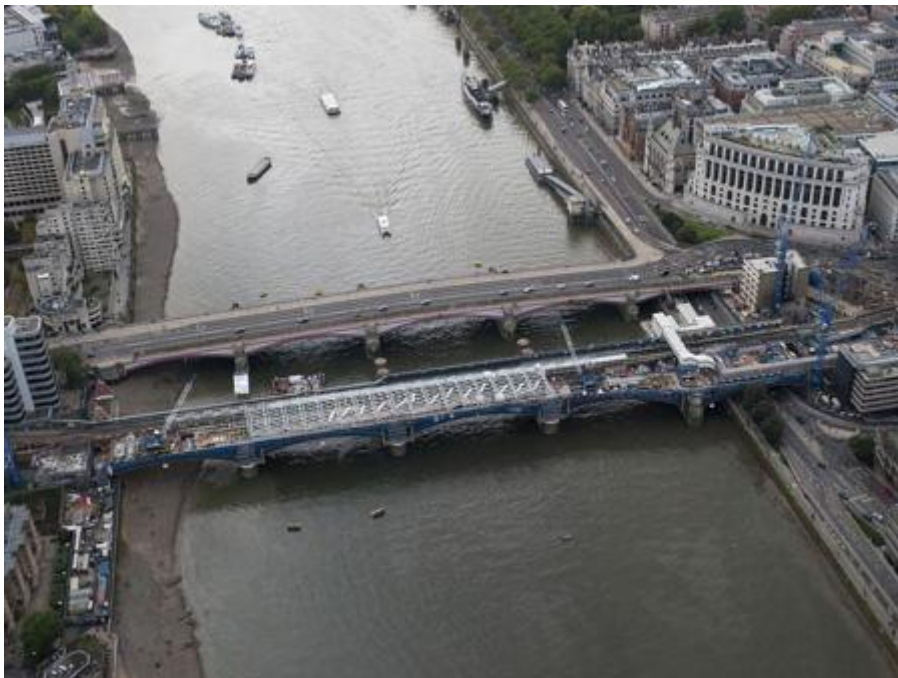
An October 2010 view of the new cross-river station at Blackfriars
