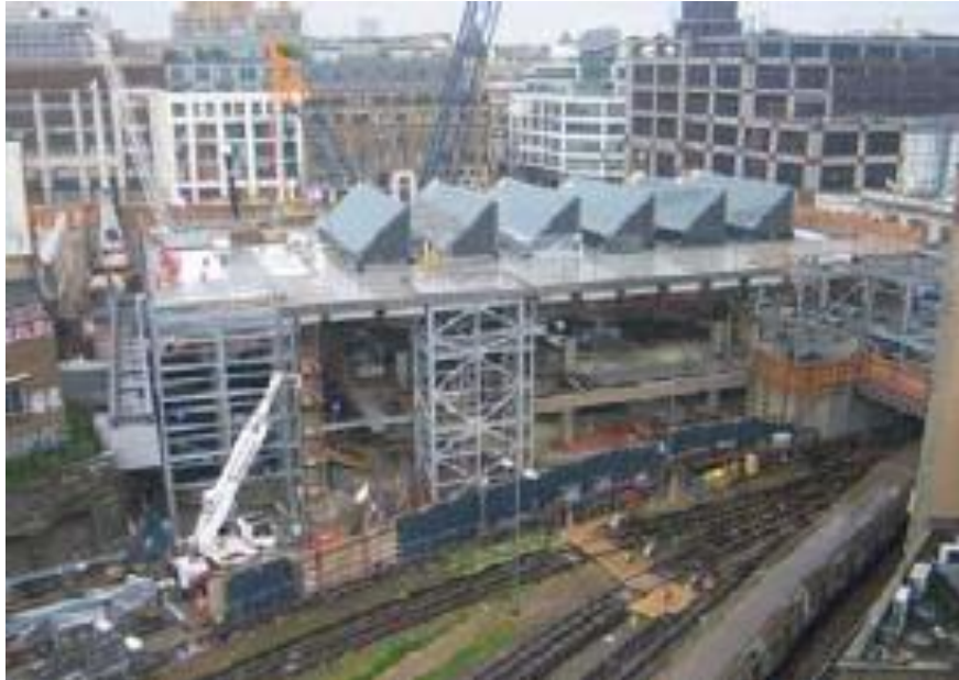
The new ticket hall at Farringdon
